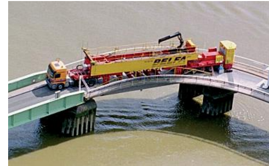
Proof loading of a bridge With the special loading vehicle Belfa
