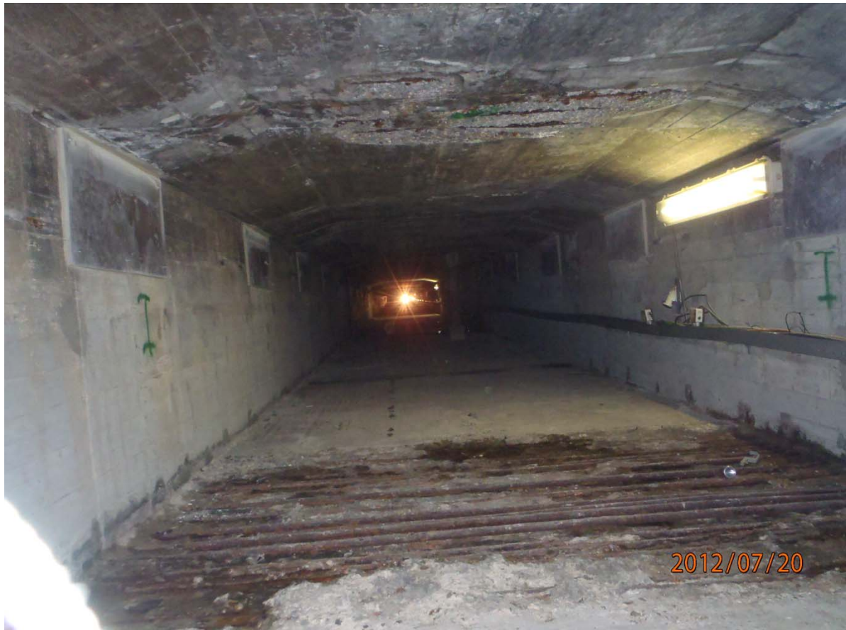
Steel bar with reduced cross section
