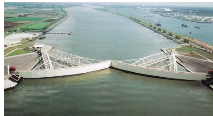
Storm Surge Barrier Hook of Holland
